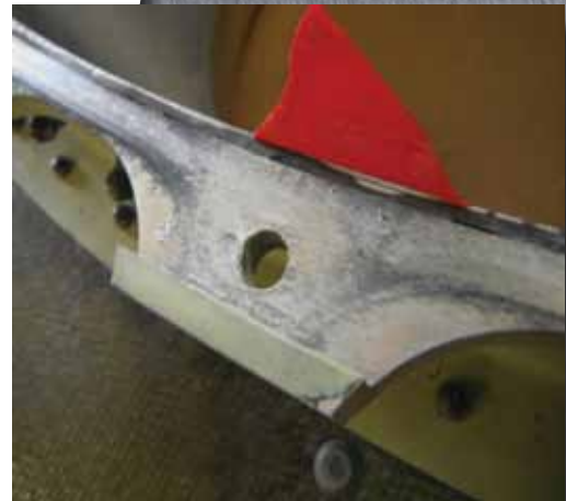
Corrosion of the Attachment Ring Mounting Holes
